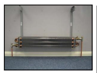
The Sovereign A Style model features a Copper Aluminium Heat Emitter, specifically designed for use within a Casing.
