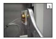
FIT THE VALVE HEAD END OF THE REMOTE TRANSMITTER TO THE BRACKET, TAKING CARE NOT TO KINK OR BEND THE CAPILLARY.
