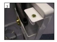
FIT THE VALVE HEAD END OF THE REMOTE TRANSMITTER TO THE BRACKET, TAKING CARE NOT TO KINK OR BEND THE CAPILLARY.
